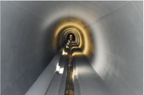
8 The Karlin cable tunnel towards the Hlávka bridge will strengthen the input from the TR Karlin to Prague 1, increasing supply reliability and freeing up the capacity of the TR Holešovice to supply developing areas in its vicinity.
