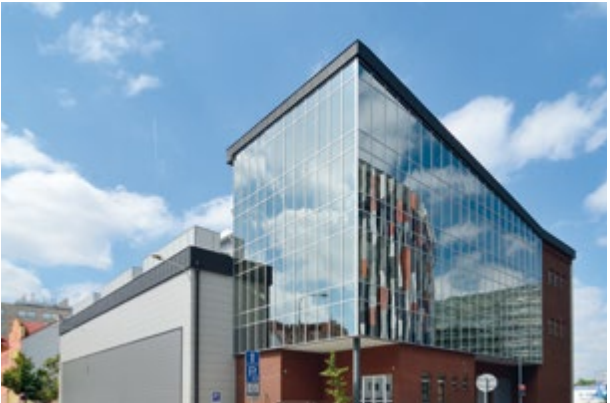
7 The new Karlin transformer station, launched in 2018, has a glass façade and an extensive green roof. The modern technological solution is practically maintenance-free and protects the roof against mechanical damage as well as weather conditions.
