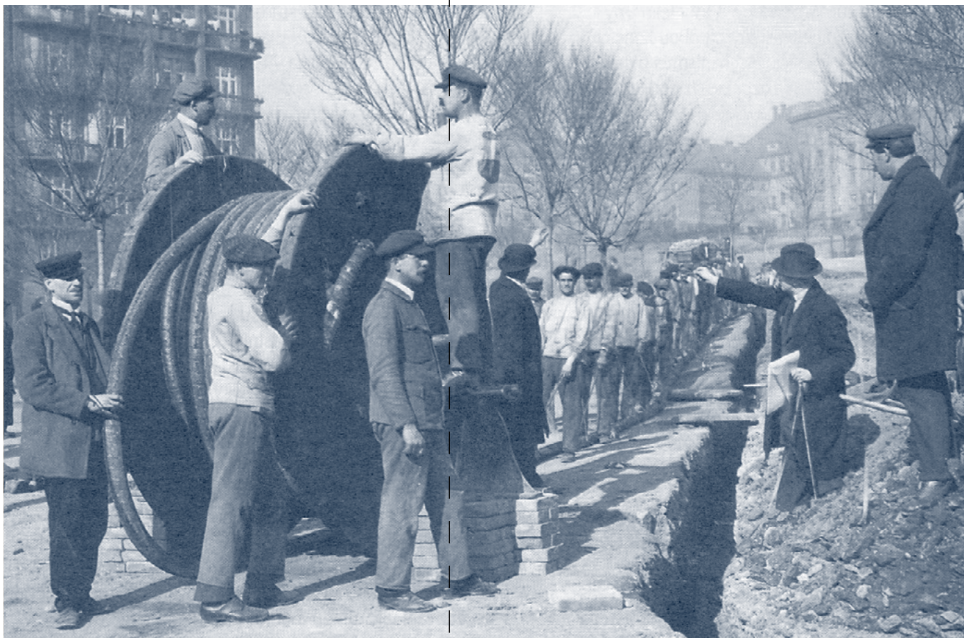
Installing high-voltage cables underground in the 1920s.
